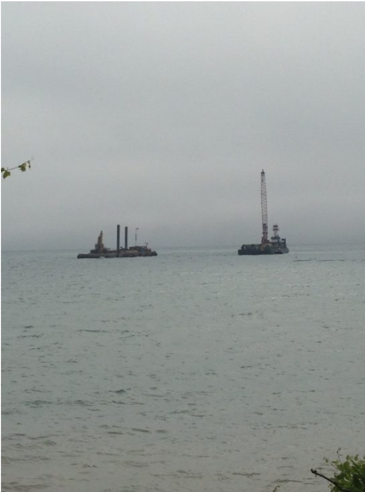
Barges situated on Lake Huron installing pipe into the lakebed.
