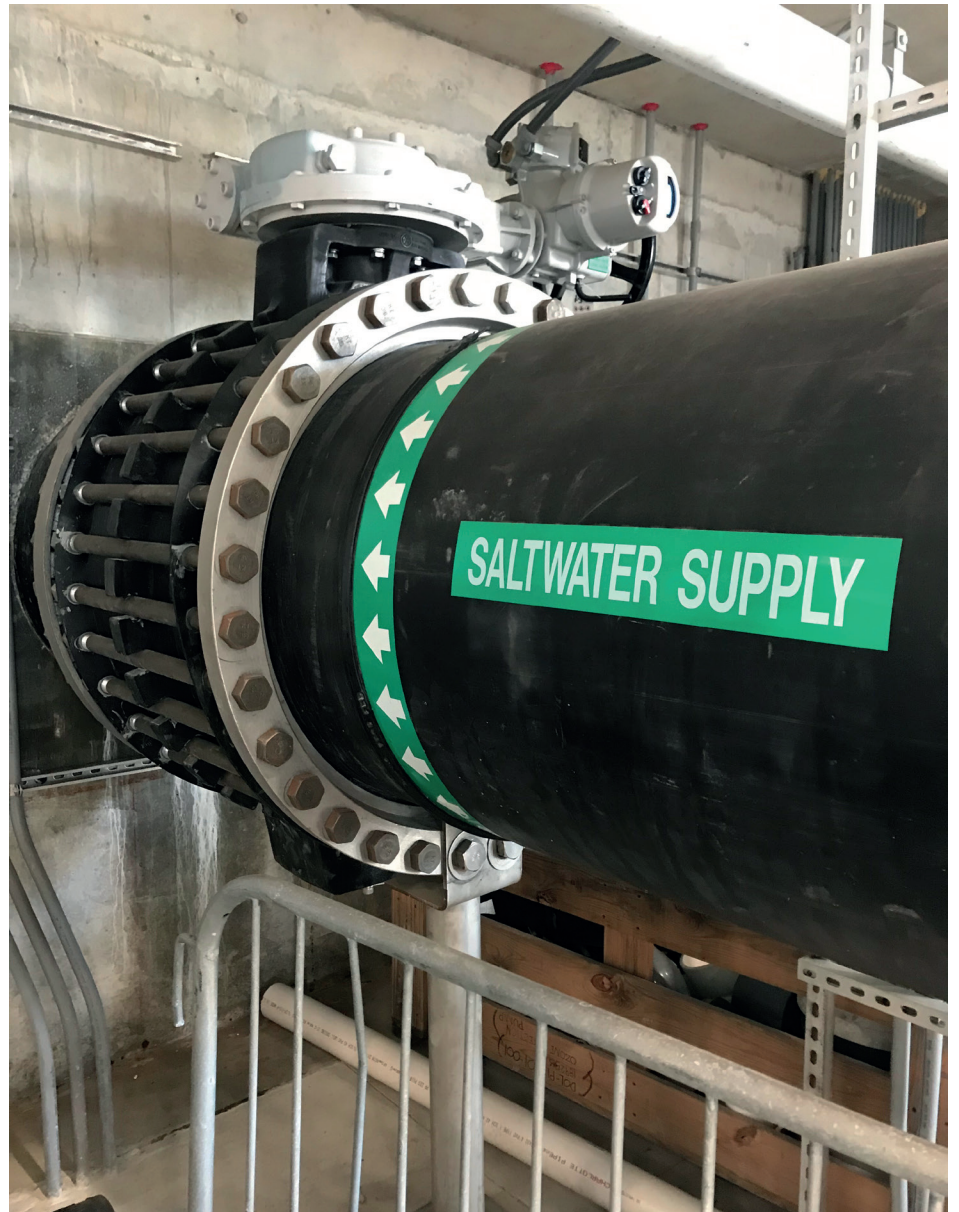
A 48" Asahi/America butterfly valve that is used on a saltwater intake line at an aquarium.
