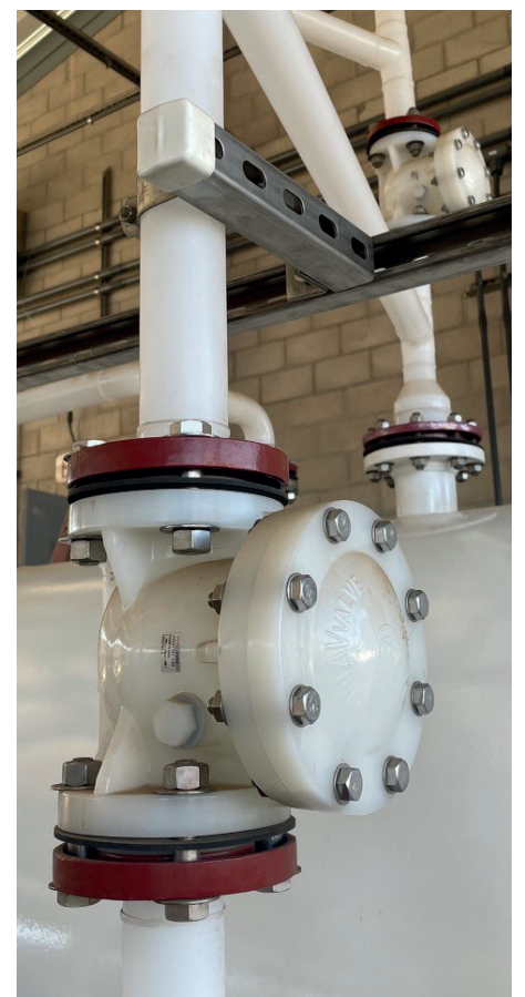
Asahi/America's PVDF swing check valve and Super Proline® PVDF piping system being used for chemical feed and filtration processes at a water treatment plant.
