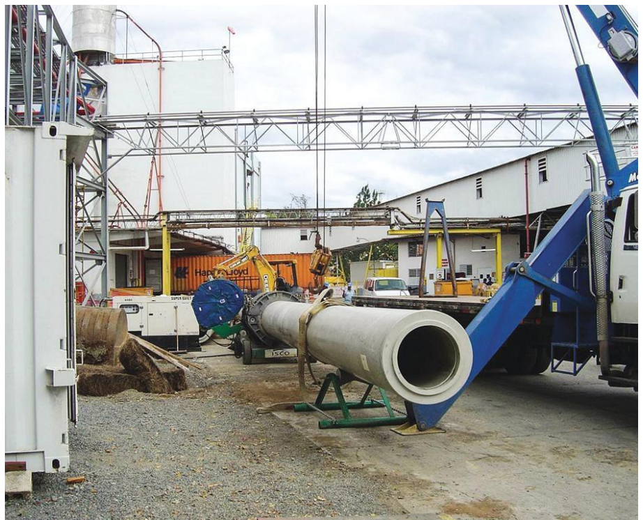
Image 1. Large diameter double-containment polypropylene system (Images courtesy of Asahi/America Inc.)
